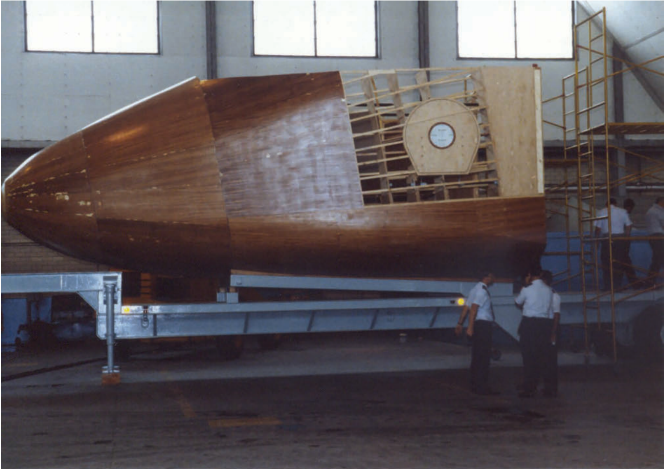
The orbiter training mockup under construction at Chanute AFB. 022 Photo courtesy of Michael Chandler
